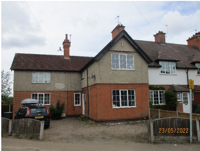
Front (north east) elevation.
